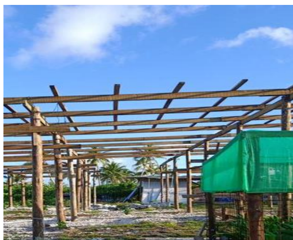
A. Shed under construction Funafala
